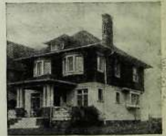
A No. 2-22-S IDEAL Boiler and 330 ft. of 38-in. AMERICAN Radiators, costing the owner $180, were used to Steam heat this cottage.
